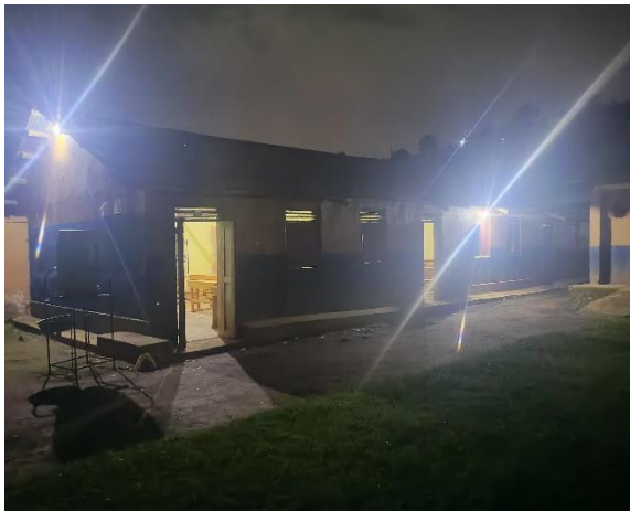
Muko High School Solar Project
